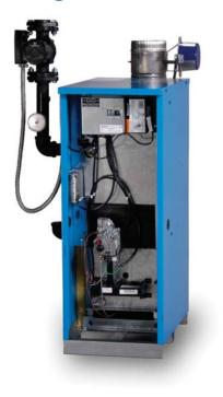
The Buderus GC124 boiler is a compact, modular boiler with all the features and benefits Buderus customers have come to expect. Designed for replacement applications, the GC124 is capable of delivering AFUE efficiencies up to 84%, with heating capacities of 74,000 thru 132,000 BTUH. All GC124 boilers are CSA approved for installation on combustible floors and are available with either standing pilot or electronic ignition.
